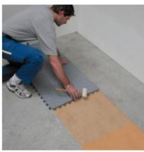
It is important that the second row is installed exactly along the chalk line.
