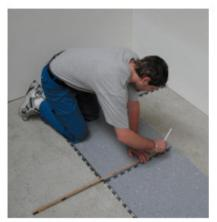
When measuring the border tiles, sufficient distance from the wall (gap) shall be allowed.
